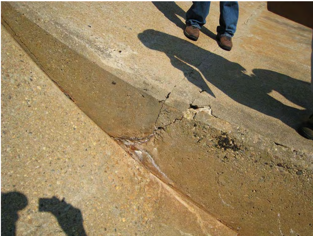
Picture on BR-S-5: Joint Between Monolith 9 and 10
