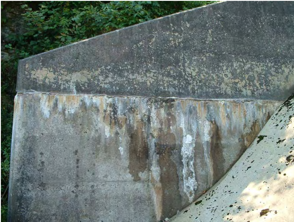
Picture on BR-S-5: Right Abutment Wall
