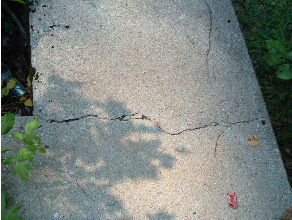
Picture on BR-S-5: Right Retaining Wall
