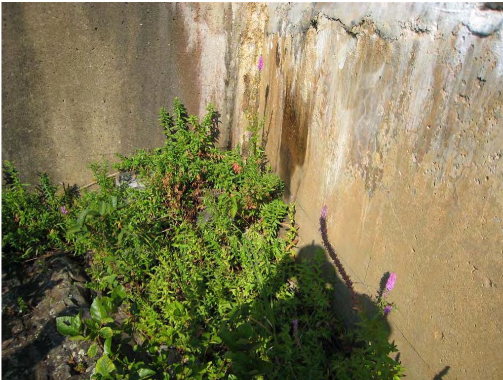
Picture on BR-S-5: Left Abutment
