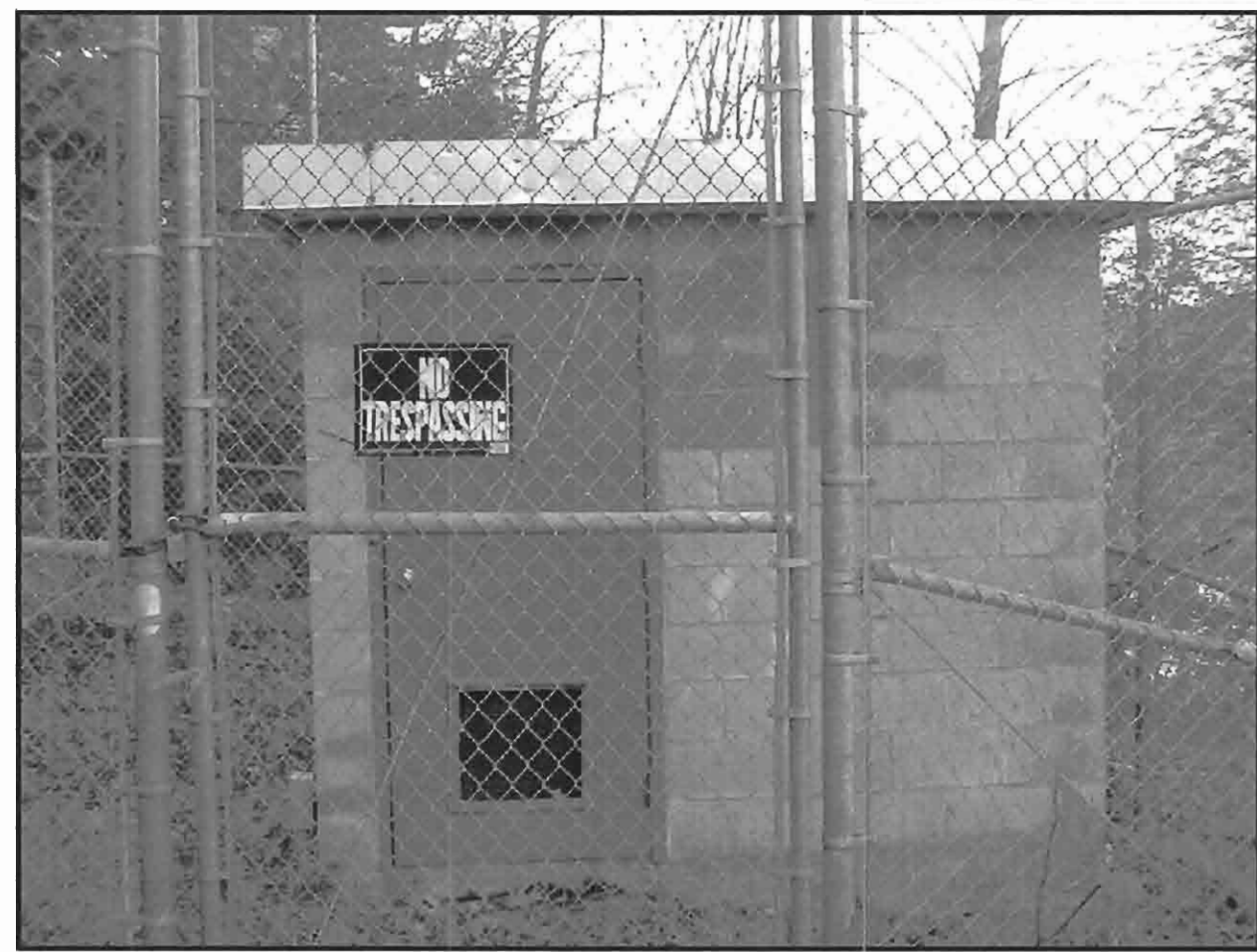
EXISTING CMU BLOCK BUILDING
