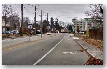
**Description**: This project includes design and construction of improvements recommended in a TEC Corridor Study. Work needed includes removal of the concrete medial islands, installation of traffic signals at the Route 1 bypass northbound ramps, re-striping to provide left turn lanes at intersections, and construction of a pedestrian refuge island at Rockingham and Dennett.
