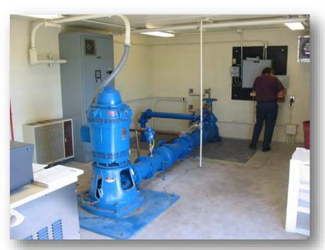
**Description**: The project consists of upgrades to existing well pump stations. The improvements include upgrades to premium efficiency motors, variable frequency drives and improvements to the radio telemetry SCADA system.
