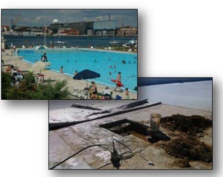
**Description**: This project includes the replacement of the pool gutter system and pool liner. The original pool was constructed in the 1930's and has been renovated a number of times. The existing liner is past the 15 year design life and the concrete gutter is starting to show signs of failure.
