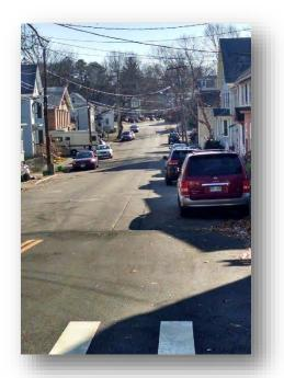
**Description**: This section of Union Street from Middle Street to State Street is in poor condition and in need of full reconstruction, streetscape improvements and full utility replacement. This will include separating the combined sewer in the area. The costs of this project will be shared with the Highway Division and Water Divisions of Public Works.
