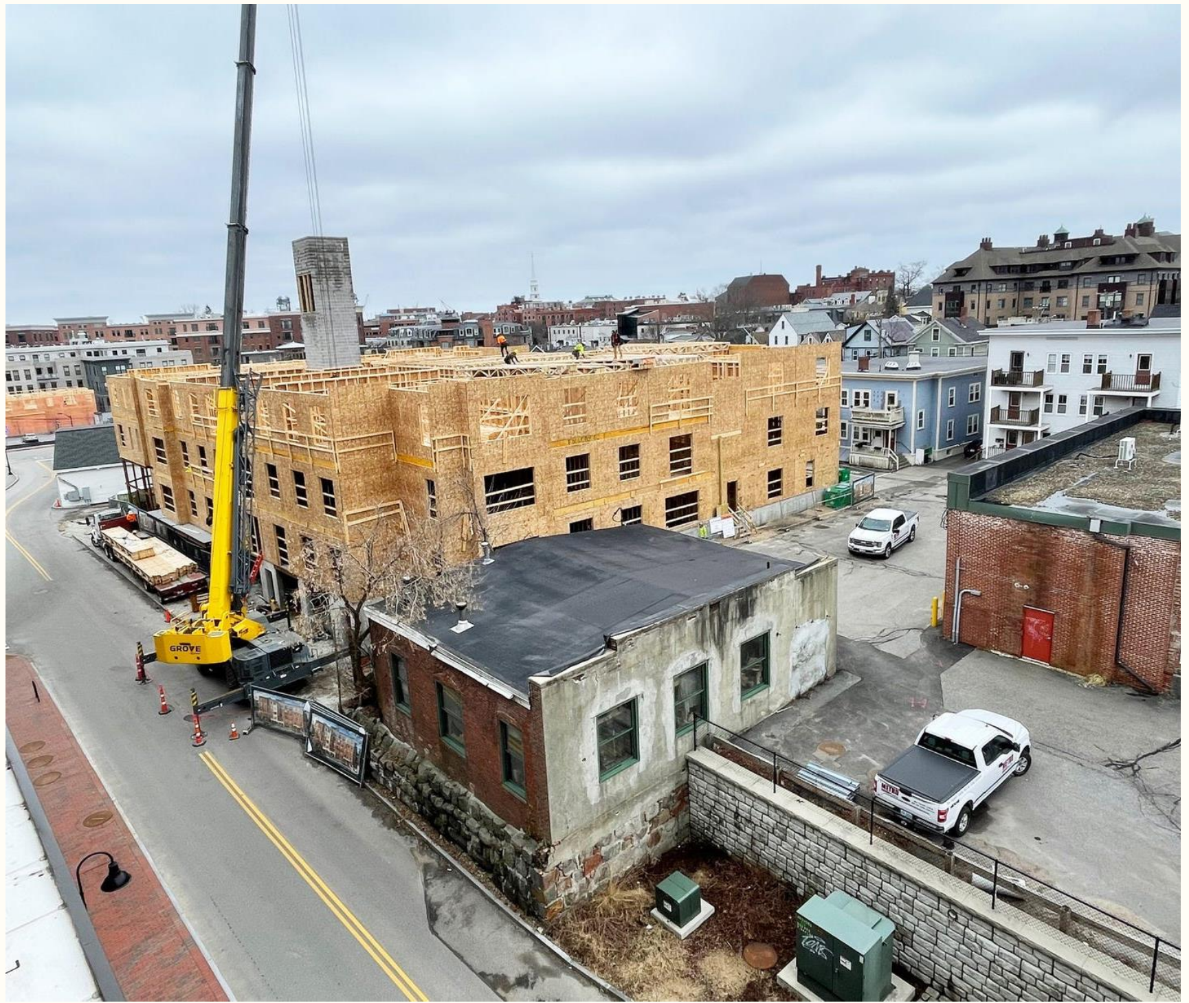
Ongoing North End construction, Seacoast Online
