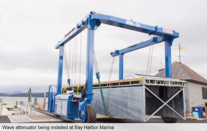
Wave attenuator being installed at Bay Harbor Marina
