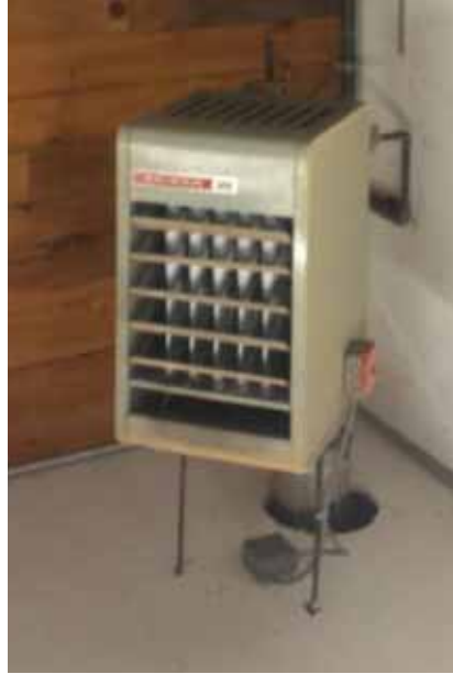
Modine unit heater serving the
