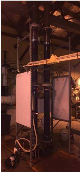
Filter 1 (left) Filter 2 (right)
