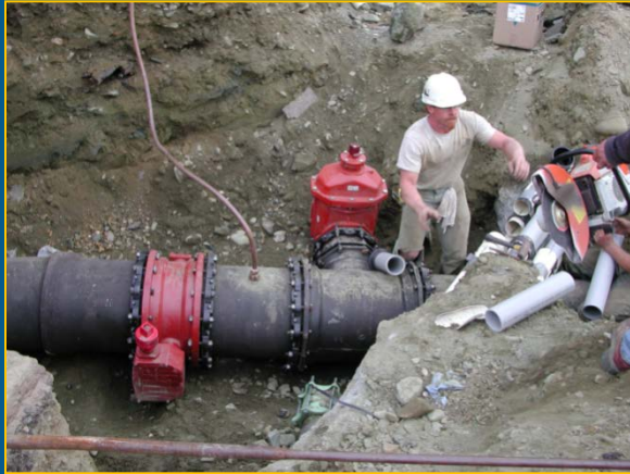
New Water Mains
