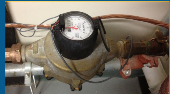
Water Meter Upgrade
