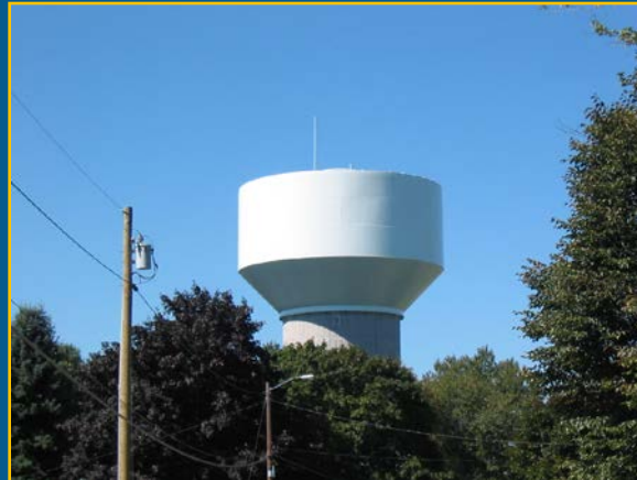
Spinney Road Tank
