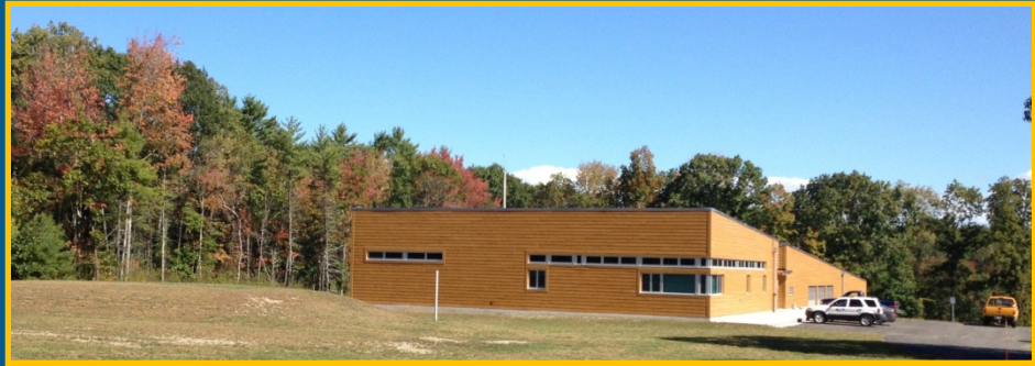
Madbury Water Treatment Facility
