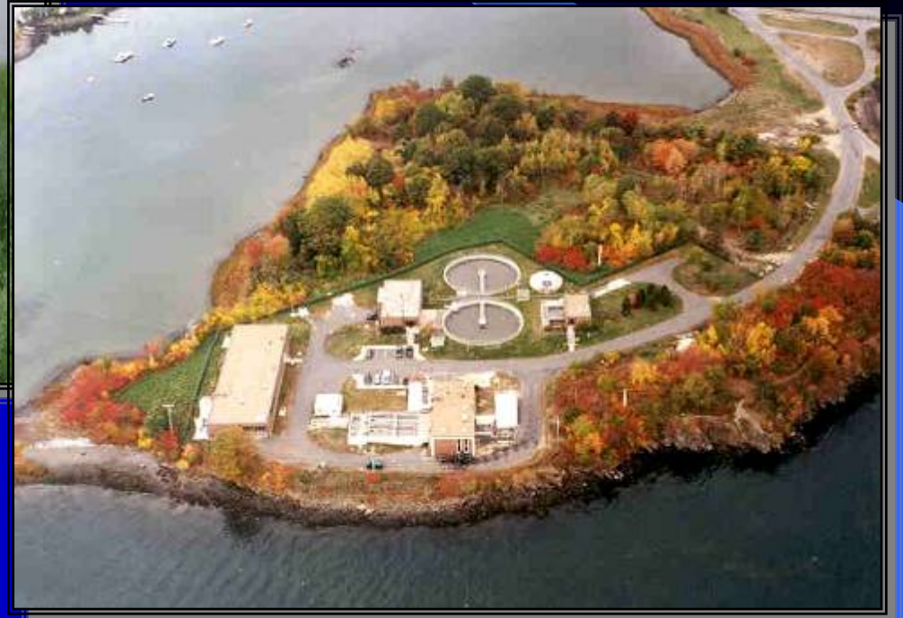
Wastewater Treatment Facilities
