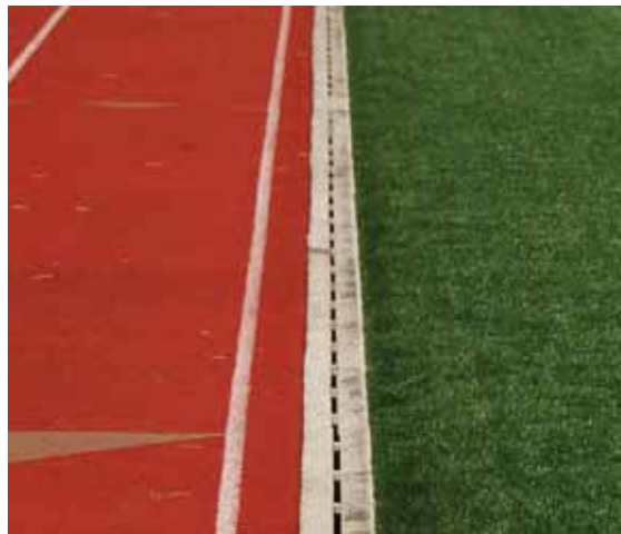
Figure 2 - Running Track Edge Drain
